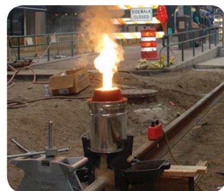
▲ The thermite process being used to join new tram lines.
