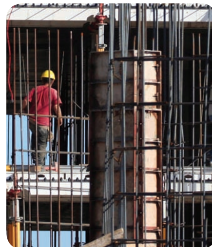
▲ Iron rods give the building strength.
